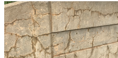
Alkali-Silica Reactivity (ASR)
